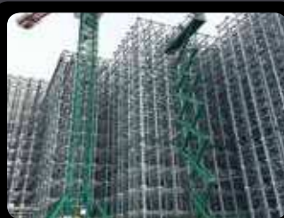
INSTALLATION INSPECTION, SERVICES
