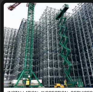
INSTALLATION, INSPECTION, SERVICES
